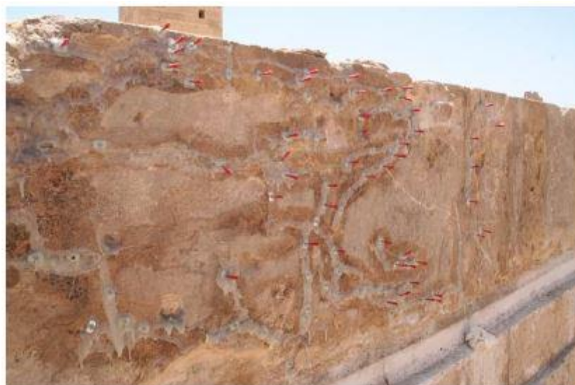
Fig. 4: The large lose part in the middles of the stone covered by hot glue. The injection channels are closed by red caps.
