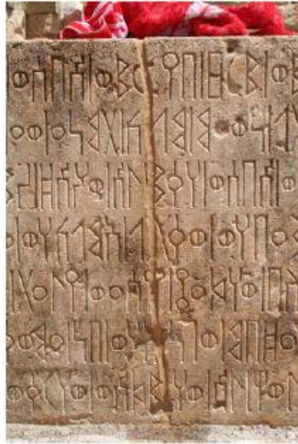
Fig. 5: The large fissure on the front site of the stone with the filling made of lime mortar.
