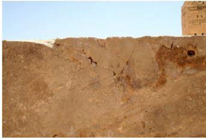
Fig. 7: The stone with the new installed broken pieces. The fissures between them and the stones are free.
